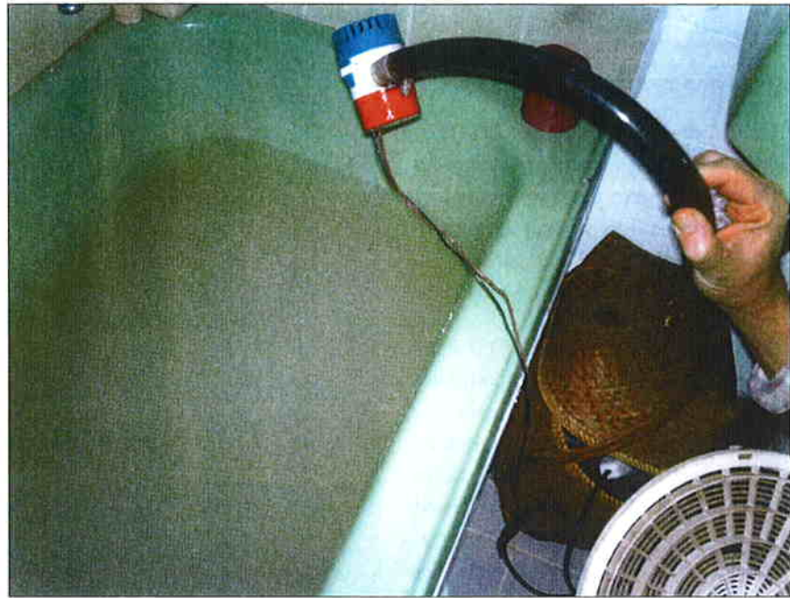
A submersible marine bilge pump is used to send water from the bath to the garden.
